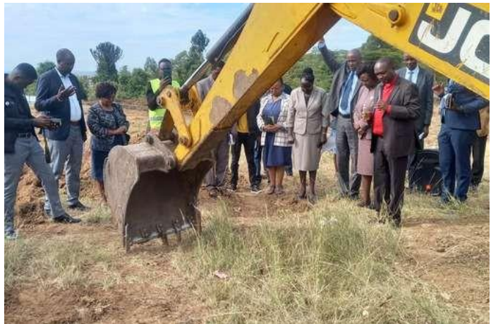
Ground breaking during the dedication
